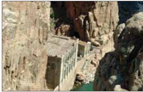
Buffalo Bill Dam, Wyo., sited on concrete, between two buildings.
