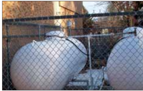
Dillon, Mont., tanks, building, sited on concrete border of sidewalk.
