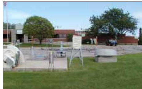
Midland, Mich., next to vent at wastewater treatment plant.
