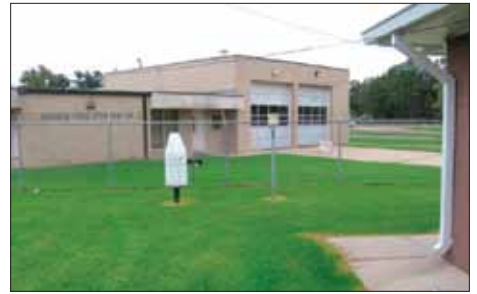
Bunkie, La., too close to sidewalk and building.
