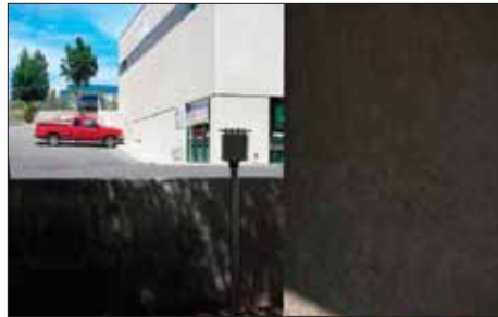
St. George, Utah, between building and raised parking lot, car radiator level.
