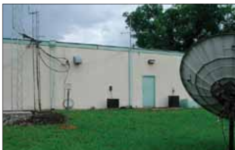
Greenville, Texas , nearby building, satellite dish, two air-conditioning units.
