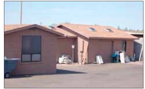
Wickenburg, Ariz., adjacent building, parking lot, accumulated junk.
