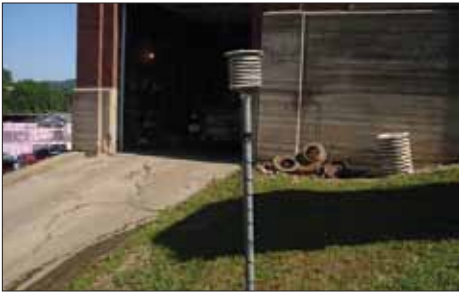
Brookville, Ind., nearby driveway, building.
