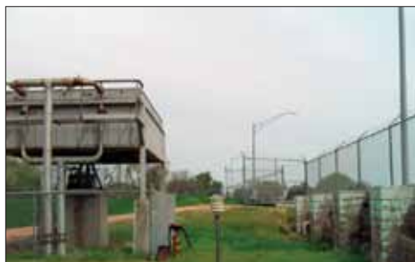
Red Cloud, Neb., on premises of city power plant. Nearby wall, structures.
